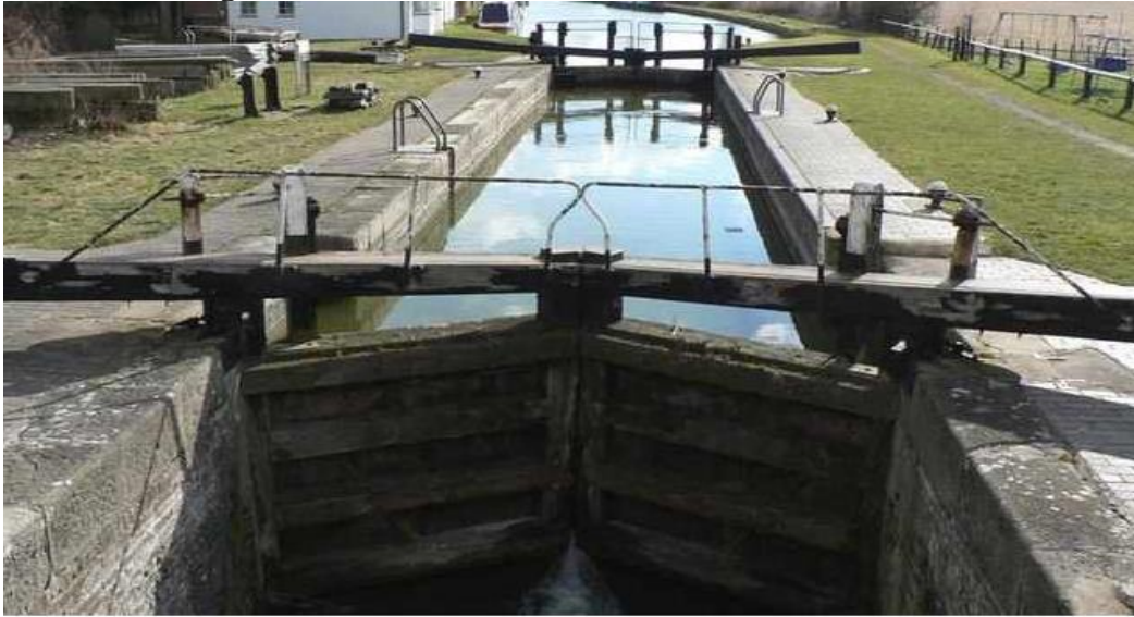
Fig-1 : Lock Gate
